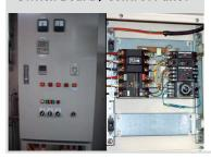
Panasonic Time Switch can be also used inside control panels as load controller.
